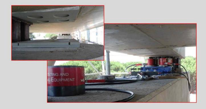
both in buildings damaged by the earthquake and in bridges and viaducts, with insertion tecnique at the base or by cutting the vertical elements of the structures.
