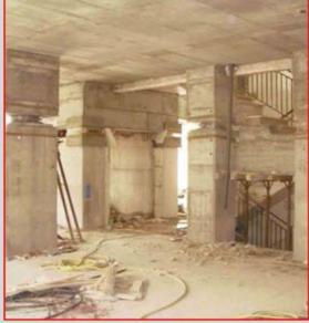
High damping ratio, obtained by using high friction coefficient for pendulum isolators and lead core for rubber isolators.
